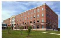
U.S. Army Legal Services Fort Belvoir, VA 33,338 sq. ft. erected in just 14 days! Architect: Perkins & Will
